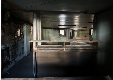
Existing below-stage partition walls and built-ins which would be reconfigured for new uses.
