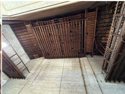
View of wood-framed grid above.
