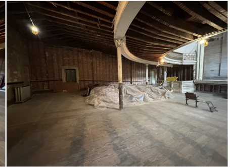
View towards house-left from the under-balcony area.
