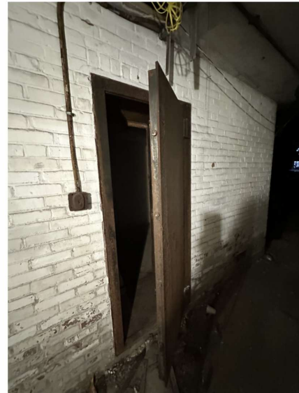
Prior jail cell in basement level.
