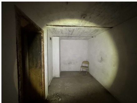
Room, at basement level, with concrete structure overhead, reinforced with steel beam.
