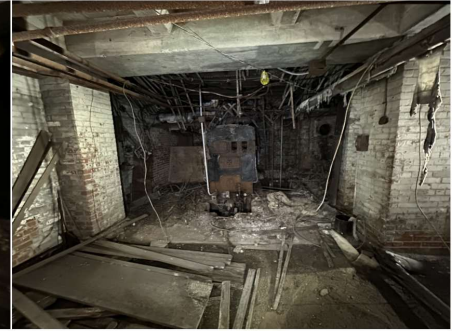
View through basement, brick pier foundations at perimeter sides, wood joist structure overhead, debris to be cleared, abated, and reused for MEP/Infrastructure.
