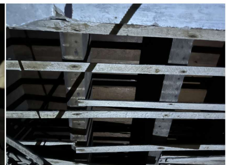
Existing wood floor structure (overhead).
