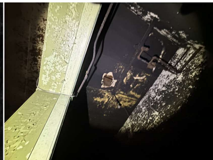
View upward to existing trap door opening in stage floor.
