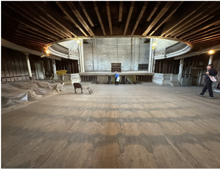
View towards stage from the under-balcony area.
