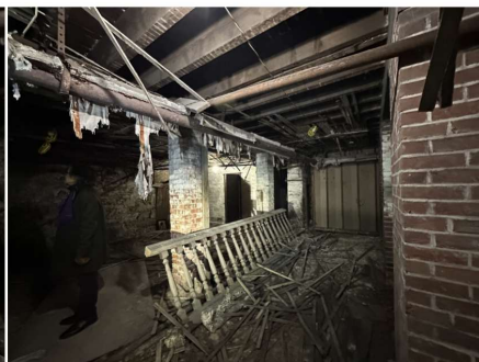
View within basement, existing brick foundation wall (beyond), wood floor joists overhead.
