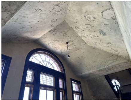
Existing plaster ceiling and exterior windows towards Elizabeth Street, lobby outside of second balcony.
