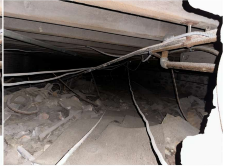
View into below-stage crawl space.
