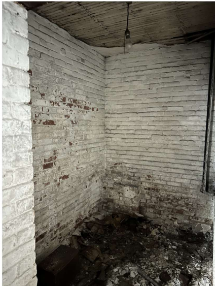
Load-bearing brick walls forming perimeter enclosure of basement room.
