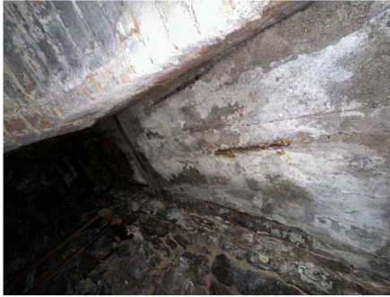
View within basement level areaway below Elizabeth street sidewalk (areaway lid overhead has since been closed).
