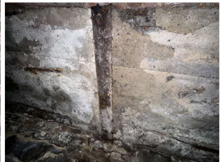
View within basement level areaway below Elizabeth street sidewalk (areaway lid overhead has since been closed).
