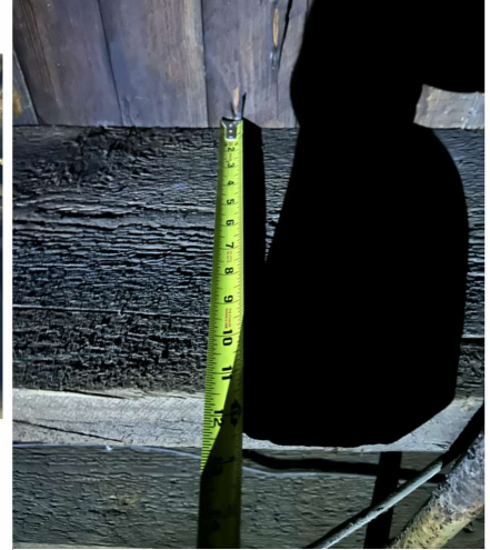
Existing wood floor joist ~11-1/2" in depth.
