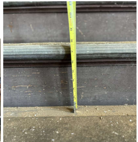
Existing lobby stair riser measurement. Lobby stairs can remain under provisions of Chapter 12 of IEBC (International Existing Building Code).
