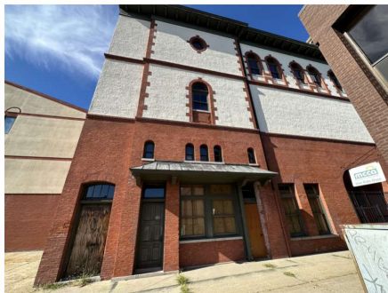
View towards southwest corner of building.
