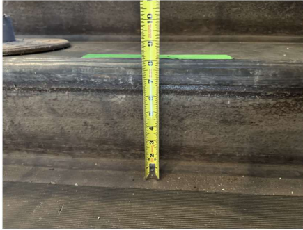
Existing lobby stair riser measurement. Lobby stairs can remain under provisions of Chapter 12 of IEBC (International Existing Building Code).
