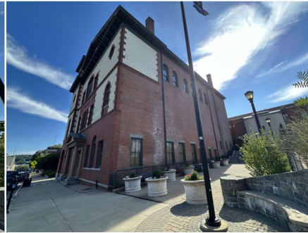
View towards north east corner of building.
