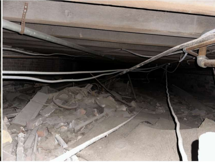
View into below-stage crawl space.
