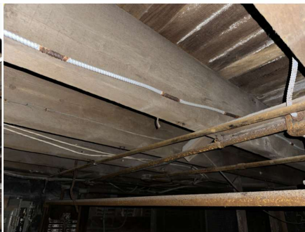
Image of wood joist structure framing the street level floor (overhead).
