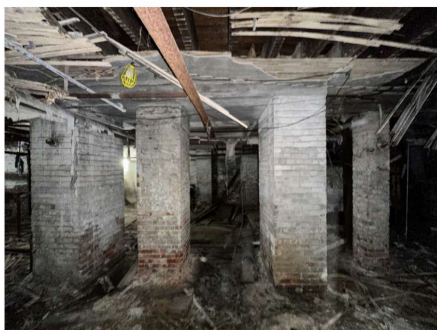
Brick foundation piers in basement.
