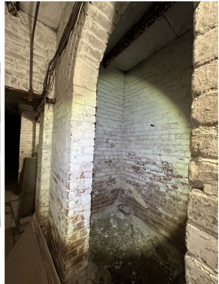
View within existing basement room. Debris to be cleared, abated, and reused for MEP/Infrastructure.
