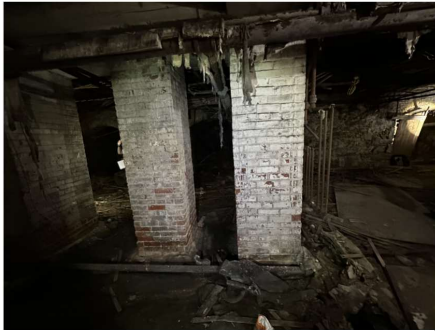
View of basement brick pier foundations.
