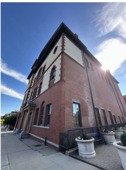
View towards north east corner of building.
