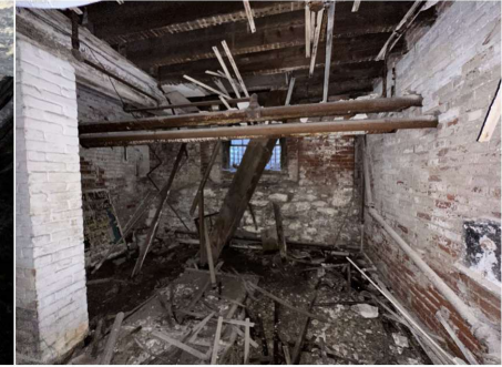
View of existing basement level stair/ladder (to be removed)
