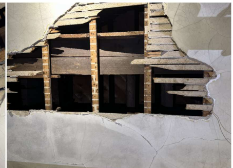
Diagonal beams framing orchestra floor above are visible through street-level ceiling.
