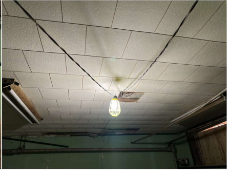
View within existing basement room. Debris to be cleared, abated, and reused for MEP/Infrastructure.
