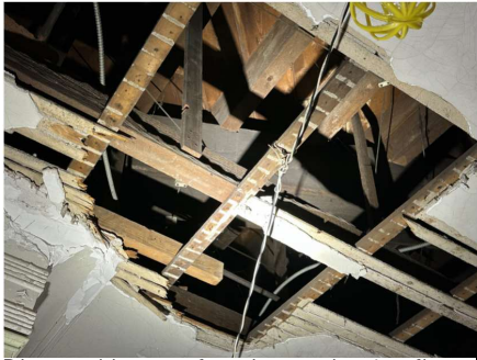
Diagonal beams framing orchestra floor above are visible through street-level ceiling.
