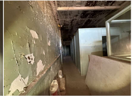
View towards existing prior half-height office partitions.
