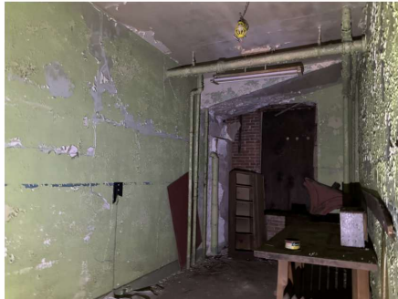
Existing street-level room.
