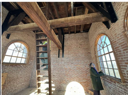
Brick perimeter walls of cupola with wood structure overhead.
