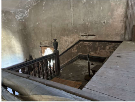
House right, rear of second balcony, looking towards balcony access stairs.
