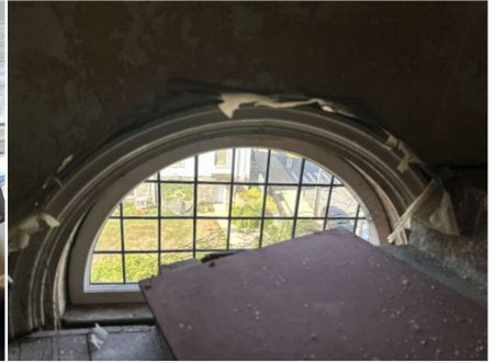
House right, rear of second balcony, existing window to exterior.
