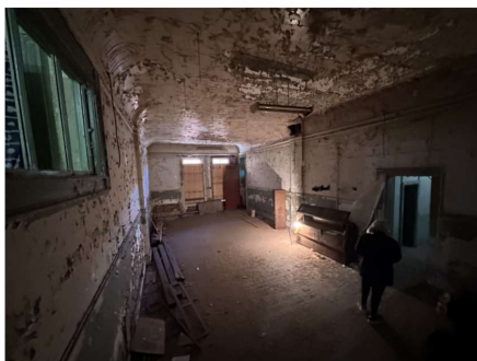
View within prior chamber room; all existing lead-based paint to be abated.
