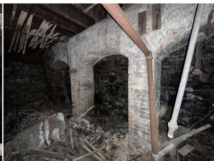
Brick archways leading to areaway in Elizabeth Street sidewalk (overhead).
