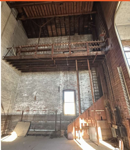
View towards stage left wood-framed fly gallery, loading gallery/grid above, and wood proscenium wall.
