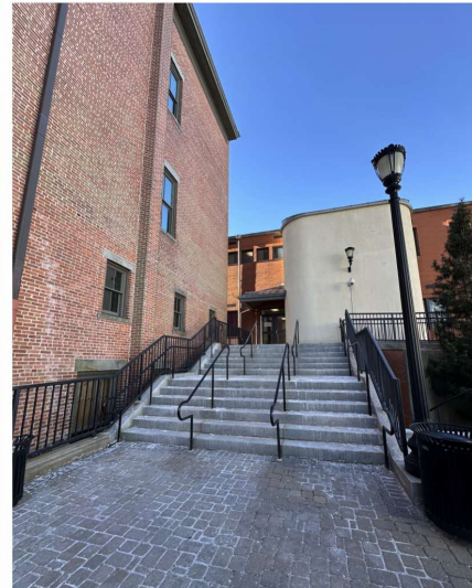
View along north side of Sterling Opera House back towards courthouse.
