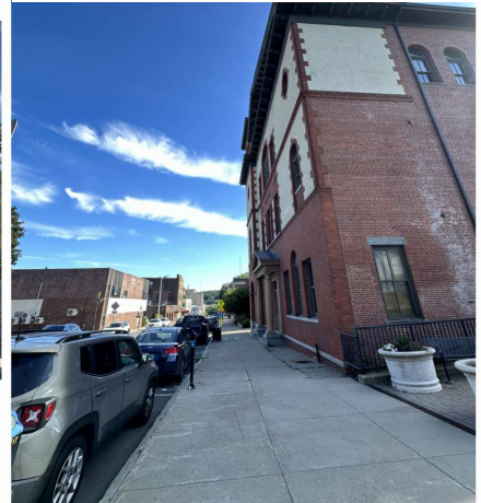
View towards north east corner of building.
