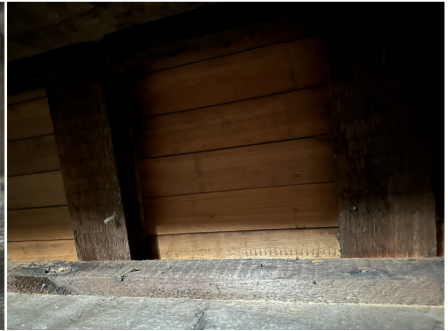
View of stage floor wood framing (overhead), stage floor planks, on wood sleepers, on wood joists.
