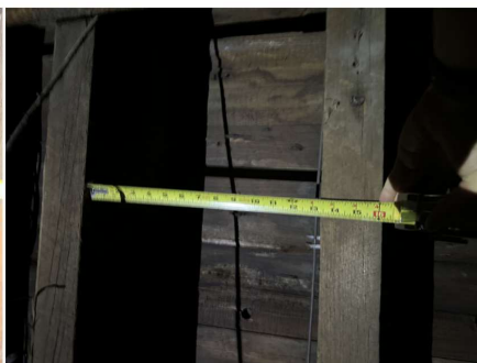
Existing wood floor joist spaced at ~16" on center.
