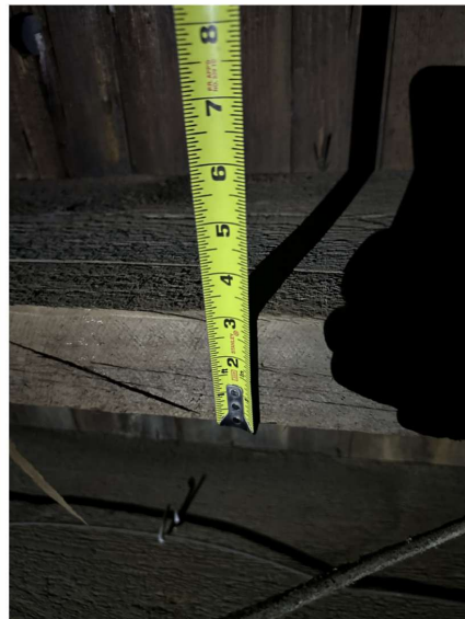
Existing wood floor joist ~3" in thickness.
