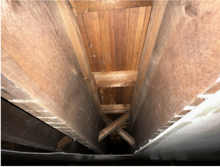
Existing wood floor joist structure of stage floor (overhead).
