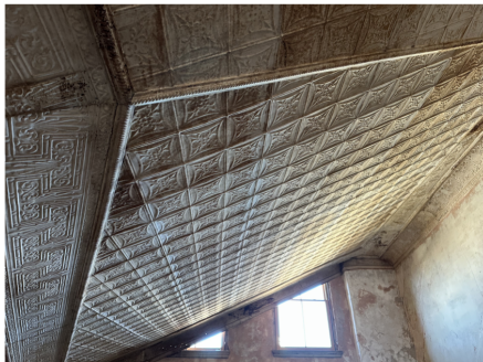
Existing ceiling at underside of second balcony.
