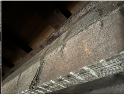
Existing wood floor joist structure of stage floor (overhead).
