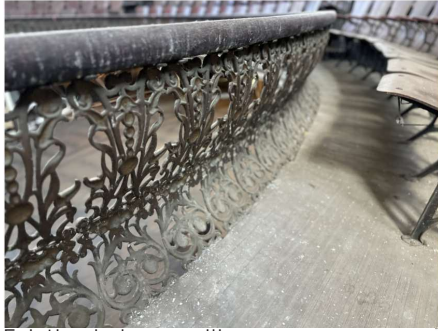
Existing balcony railing.
