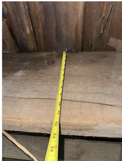
Existing wood floor joist ~12" in depth.
