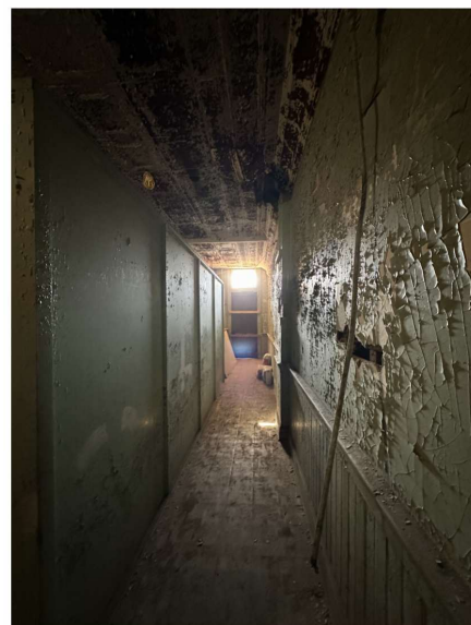
View down below-stage street level corridor.
