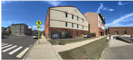
View looking north on Olivia Street at end of what could be loading drive towards the Sterling.
