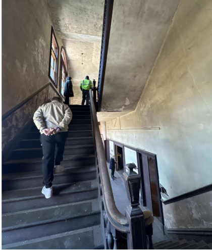
Image of existing lobby stair.
