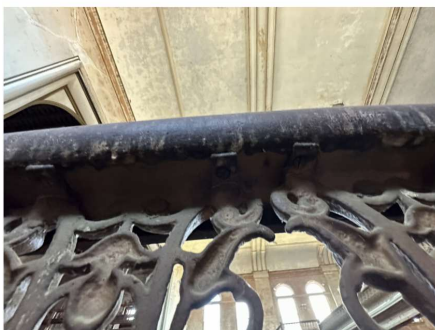
Existing balcony railing.
