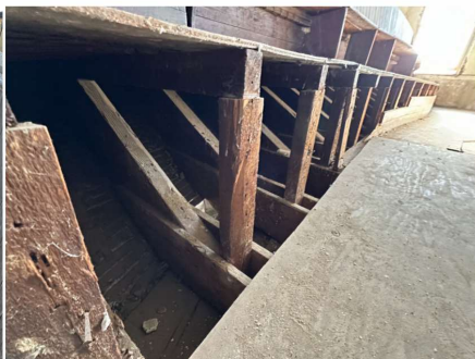
Existing wood framing of second balcony tiers, to be replaced.
