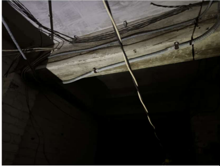
Wood beam supporting wood joists overhead, spanning between brick columns in basement.
