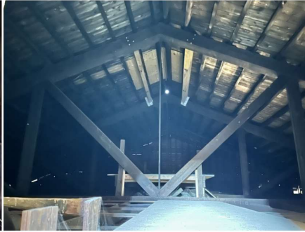
Heavy timber roof trusses span over the audience chamber.
