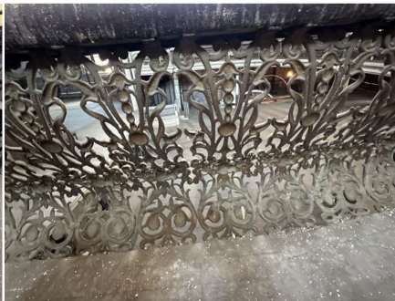
Existing balcony railing.
