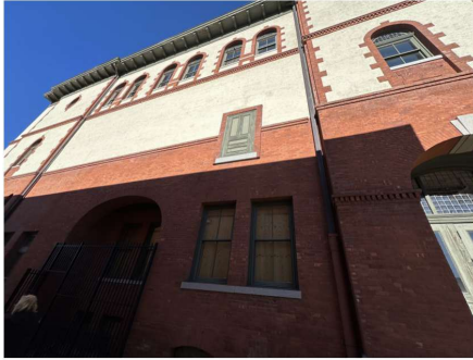
View towards south side of building.
