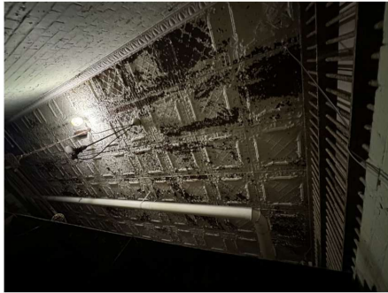
Ceiling of prior jail cell room
