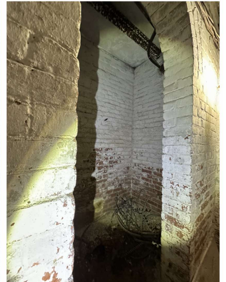
Room with brick perimeter walls in basement.
