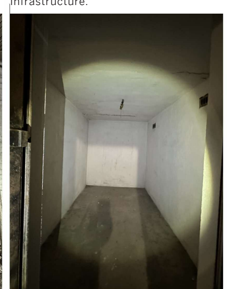
View within safe room.
