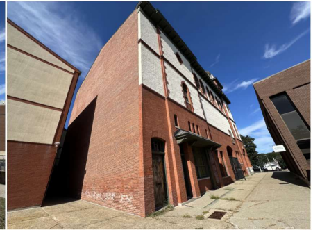
View towards southwest corner of building.
