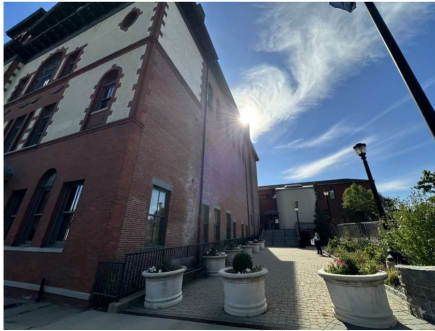
View towards north east corner of building.
