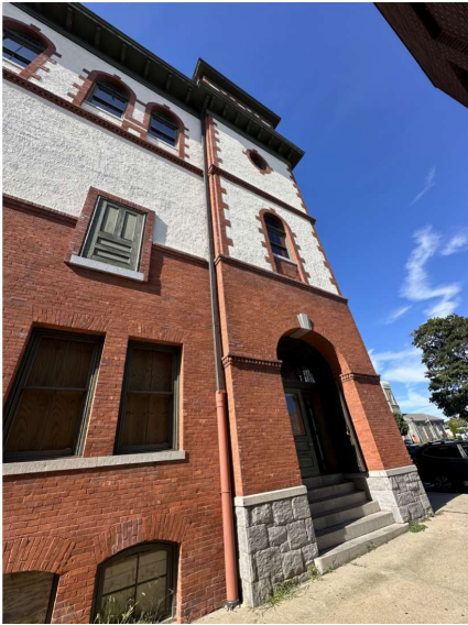
View towards south side of building.
