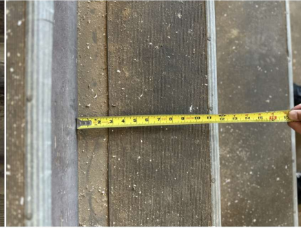
Existing lobby stair riser measurement. Lobby stairs can remain under provisions of Chapter 12 of IEBC (International Existing Building Code).
