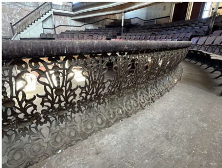
Existing balcony railing.
