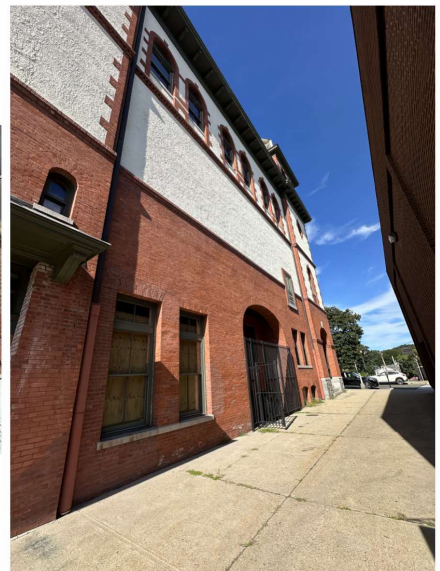
View towards south side of building.
