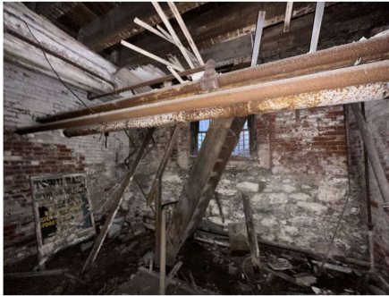
View of existing basement level stair/ladder (to be removed)
