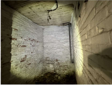
Room with brick perimeter walls in basement, existing wood lath overhead.
