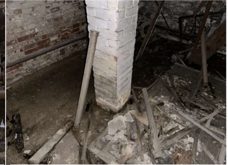
Brick column termination at basement floor.
