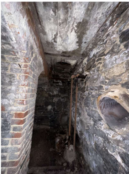
View within basement level areaway below Elizabeth street sidewalk (areaway lid overhead has since been closed).
