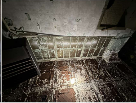
Prior chamber room ceiling.
