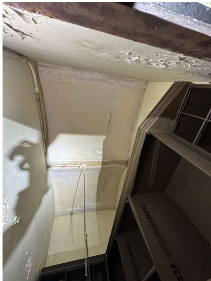
Existing plaster ceiling of street-level room.
