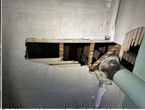
Existing cast iron column at street level continues structural load of balconies (above) down to foundations (below).
