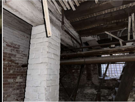
Brick column in basement, supporting beam overhead.
