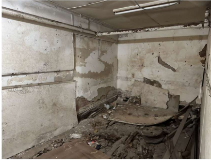
View within existing basement room. Debris to be cleared, abated, and reused for MEP/Infrastructure.
