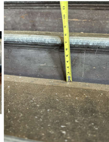
Existing lobby stair riser measurement. Lobby stairs can remain under provisions of Chapter 12 of IEBC (International Existing Building Code).
