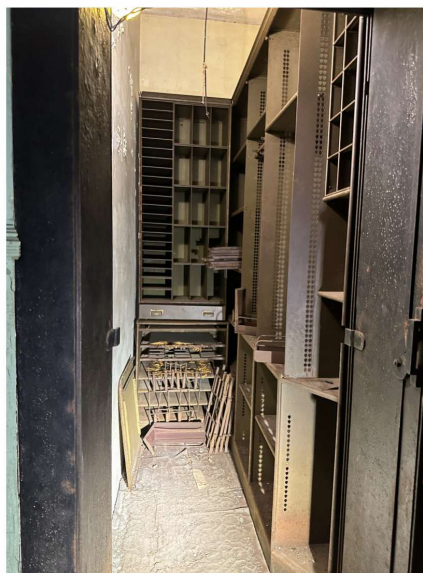
View into prior street-level safe room.
