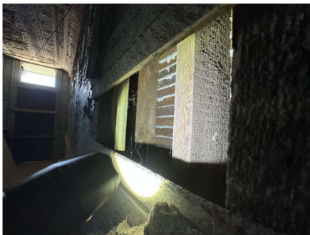
View within street level room of make-up of existing plaster partition wall.
