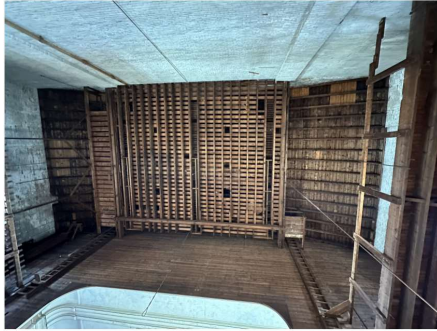
Wood framing of existing stage grid.
