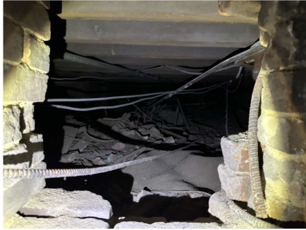
View into below-stage crawl space.
