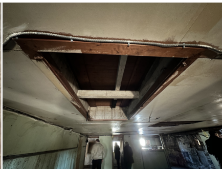
View of prior stage trap opening (overhead) into below-stage level.
