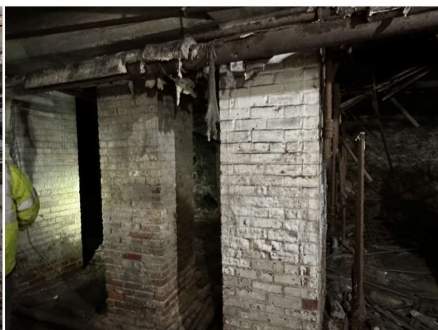
Brick foundation pier in basement.
