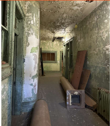
View down corridor upon entry at street level off of Elizabeth Street. Many street level partitions will be removed and reconfigured. All existing lead-based paint to be abated.
