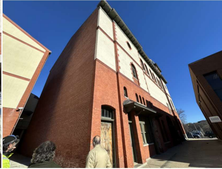
View towards southwest corner of building.
