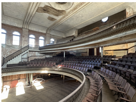
View from house left side of first balcony back towards second balcony.
