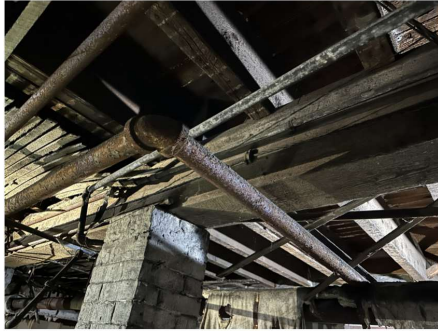
View from basement below to wood joist floor structure (overhead). Existing sprinkler (non functioning) overhead.
