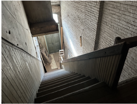
Existing exit stair from below-stage level to street.
