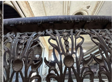
Existing balcony railing.
