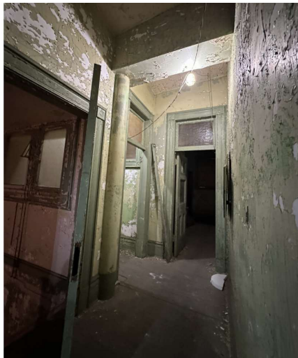
Interior view from street-level corridor towards prior men's and women's restrooms.
