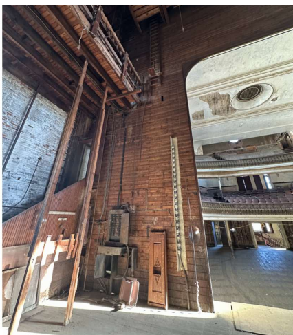
View towards stage left proscenium wall.
