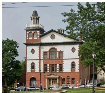
View towards main facade (east façade) of building.
