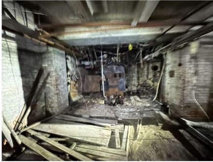
View through basement, brick pier foundations at perimeter sides, wood joist structure overhead, debris to be cleared, abated, and reused for MEP/Infrastructure.
