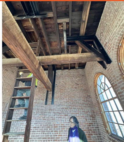
Brick perimeter walls of cupola with wood structure overhead.
