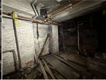
View of basement brick foundation walls, wood joist structure overhead, existing plumbing/fire protection piping (non functional) overhead.
