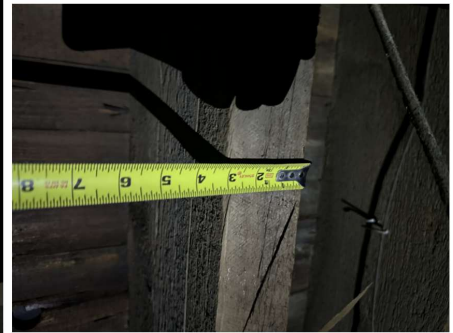
Existing wood floor joist ~3" in thickness.
