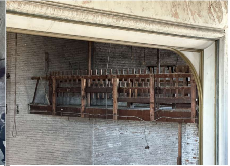
Close-up view from audience towards stage left fly gallery, pin rail, and wooden belaying pins.
