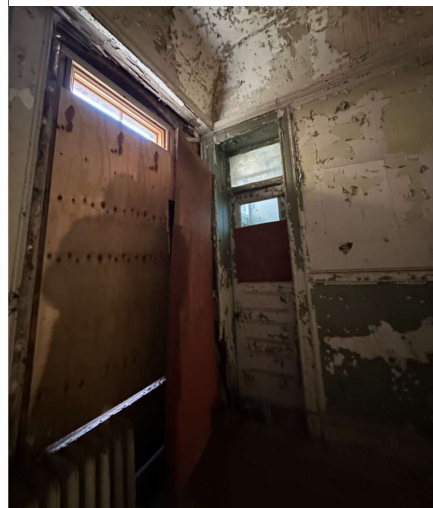
View within prior chamber room; all existing lead-based paint to be abated.
