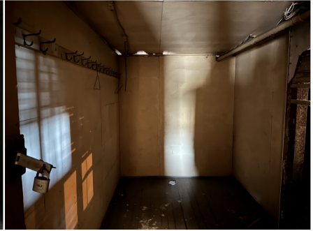
Existing below-stage partition walls and built-ins which would be reconfigured for new uses.
