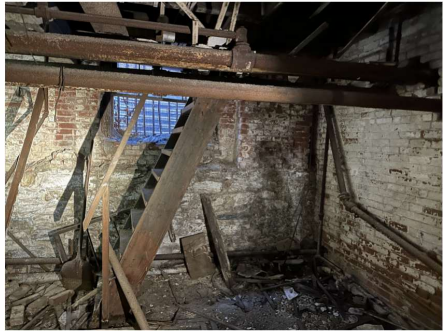
Existing ladder/stair to street level
