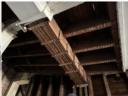
Wood framing below balcony, including wood joists on laminated wood beam structure.
