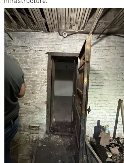
View of safe room door (from exterior side).
