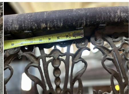
Existing balcony railing is formed out of modular cast iron sections about ~7-inches in width allowing for easy replication or replacement of individual sections.
