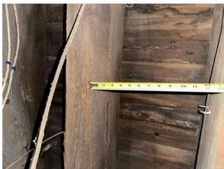
Existing wood floor joist spaced at ~16" on center.
