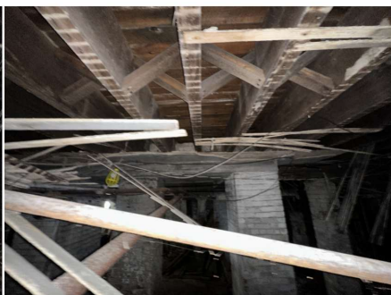
Wood joist floor structure (overhead); brick foundation piers beyond.
