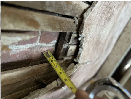
Thickness of plaster wall make-up.
