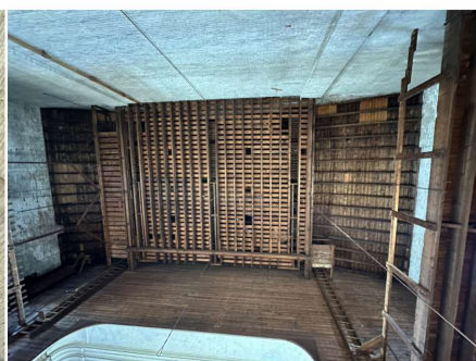
View of wood-framed grid above.
