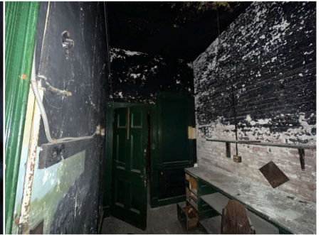
View into prior office at street level.
