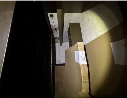
View into prior street-level safe room.
