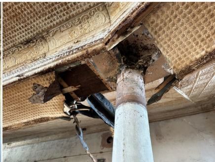
Existing ceiling and structure at underside of second balcony.
