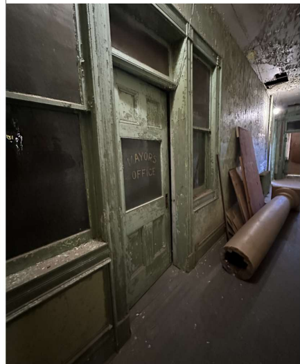
View down central street level corridor, looking towards prior mayor office.
